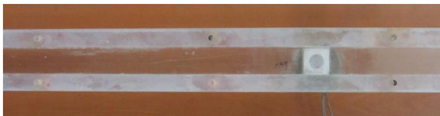
Fig5. Top view of a part of the channel
